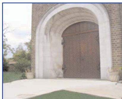
St Anselms Church after access improvement work
