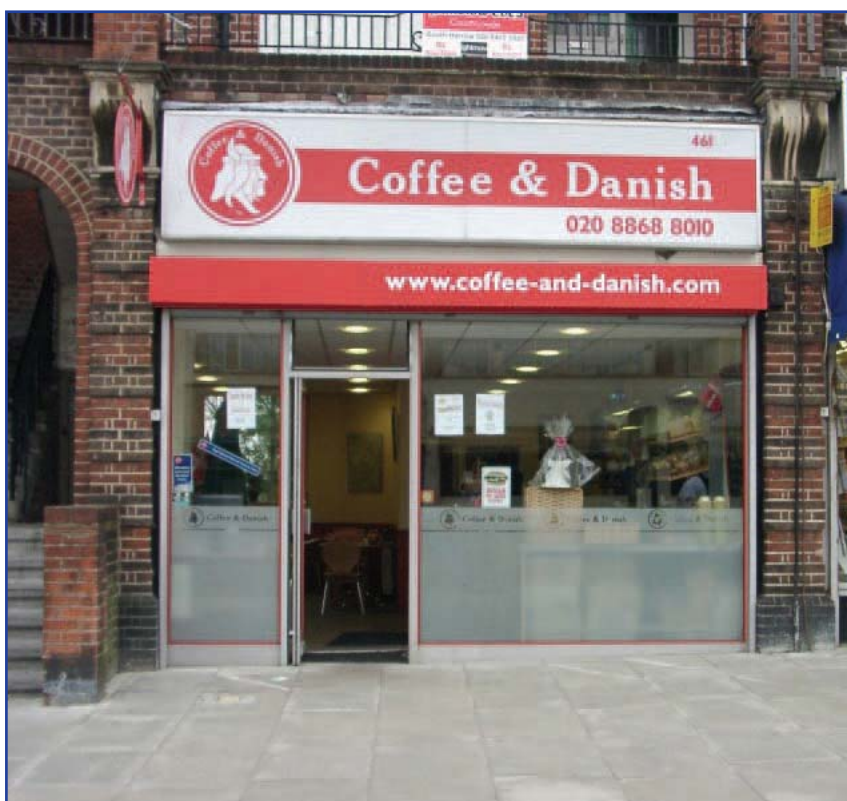
Option 1:- Accessible threshold
