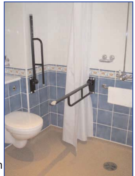
Accessible ensuite bathroom with 'wet floor' shower facility
